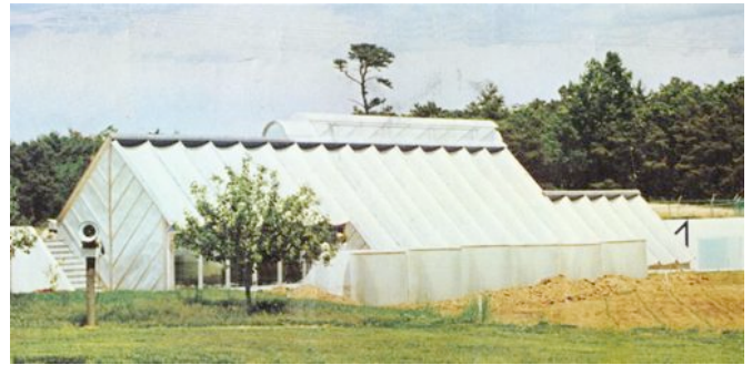
1976 original Ark structure -
